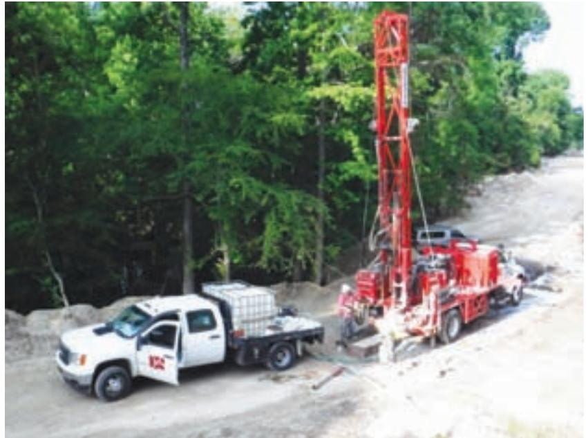
remedial measures for these two bridges. D&S mobilised its 2015 Mobile B-57 truck-mounted drilling rig for both sites.
